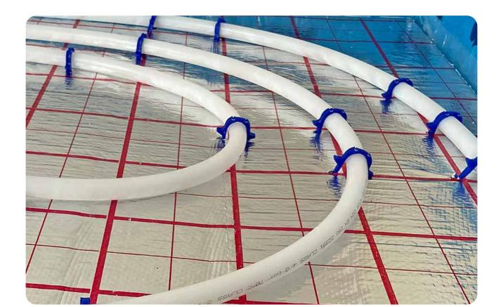
**PRL** and **PRL HP** are traditional underfloor heating and cooling systems, characterized by pipe anchored to the insulated base and embedded in the screed.
