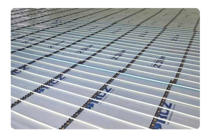
**PVC bar** system is a solution for underfloor heating in industrial buildings characterised by pipes housed in a support bar anchored to an insulating panel base.
