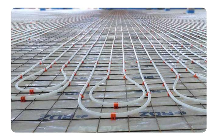
**Industrial mesh** system is a solution for underfloor heating in industrial buildings characterised by piping anchored to the mesh by special clips and embedded in the screed.
